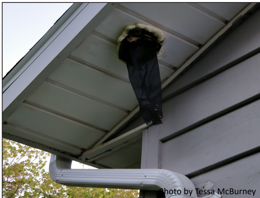
Figure 16. One-way eviction device in place for an exclusion.
